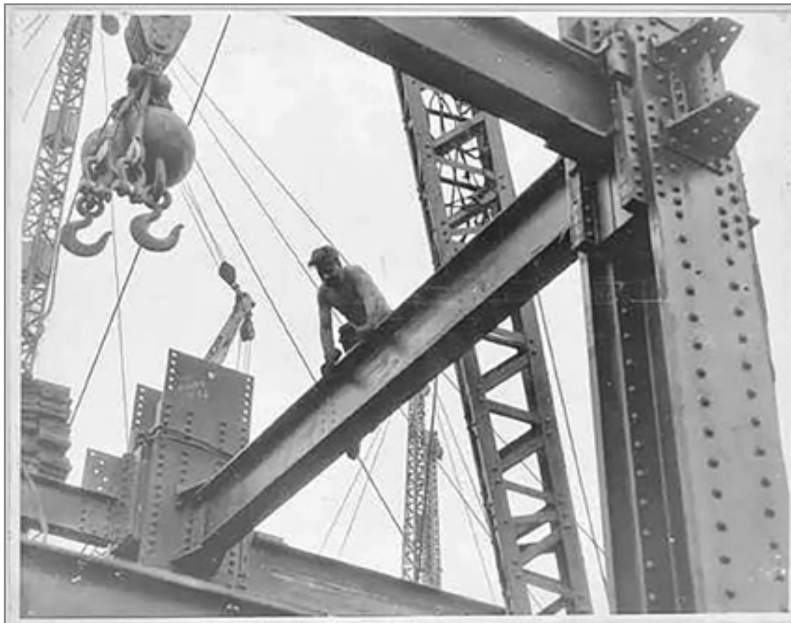
Travi e operai, Empire State Building 1930-1931
