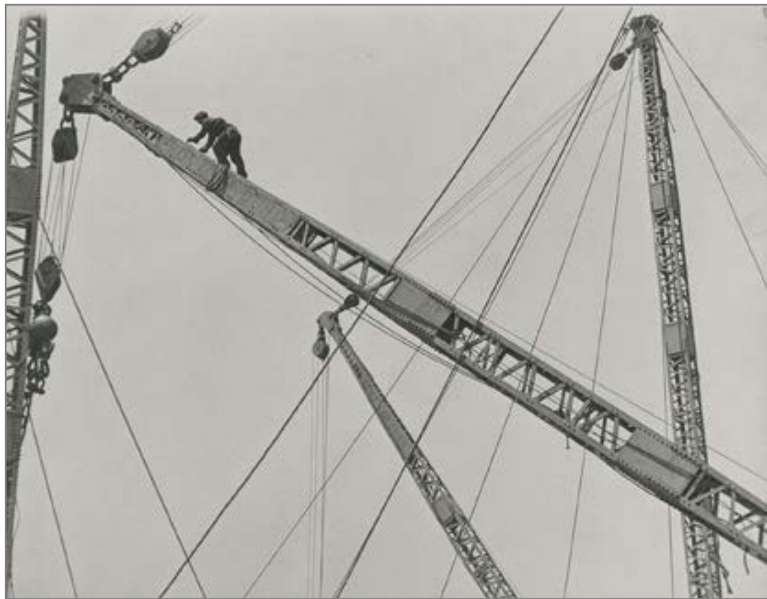
Gru a traliccio, Empire State Building, New York, circa 1930
